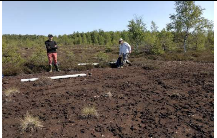
Figure 3.1.4. Installation of the water level monitoring well Cena4 in the degraded part of the Cena Mire, PeatCarbon restoration site, June 8, 2023. Image: © A. Kalvāns
