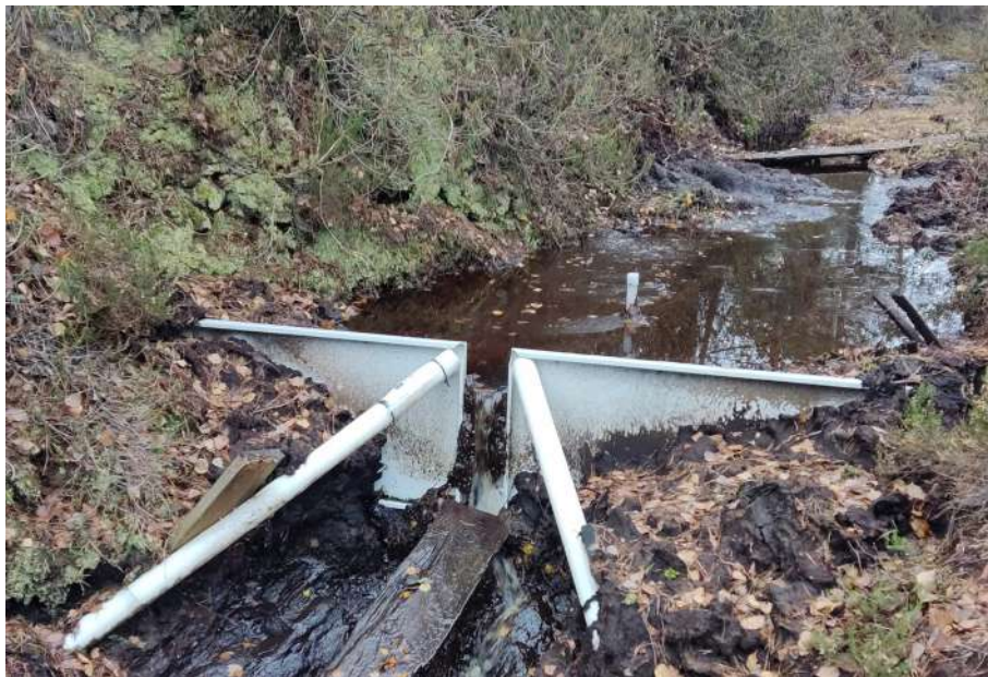
Figure 3.1.9. A discharge measurement spillway (monitoring point Cena8) clogged with eroded peat, November 10, 2023. Image: © A. Kalvāns
