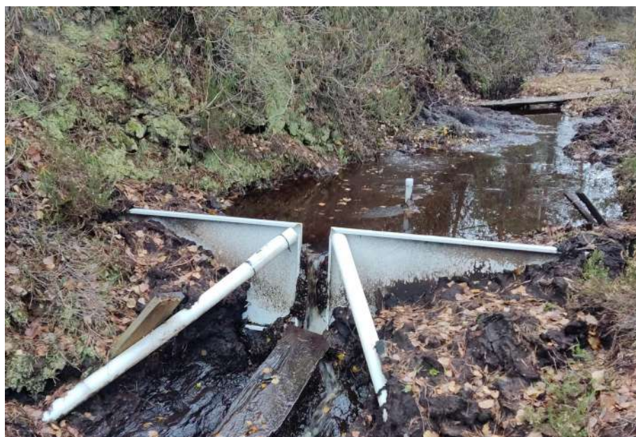
Figure 3.1.16. A discharge measurement spillway (monitoring point Cena8) clogged with eroded peat, November 10, 2023. Image: © A. Kalvāns
