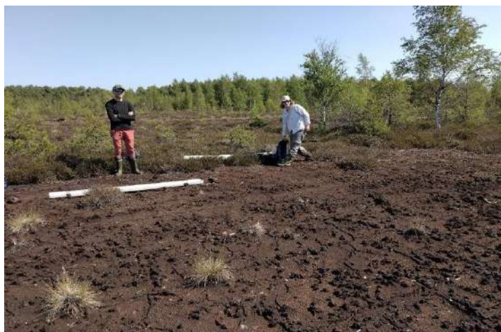
Figure 3.1.11. Installation of the water level monitoring well Cena4 in the degraded part of the Cena Mire , PeatCarbon restoration site, June 8, 2023. Image: © A. Kalvāns
