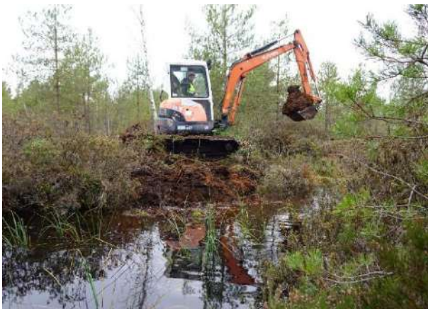
Figure 1.1.3. On the left: dam building in Cena Mire in autumn 2025. On the right: participants of a demonstration seminar stand on a newly completed dam after observing the dam-building process. Images: © L. Strazdiņa, R. Gorodko
